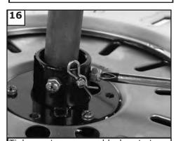
Tighen set screws and lock nuts to secure downrod in place.
